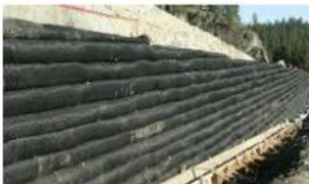
Figure 1: Typical wrapped face MSE walls
